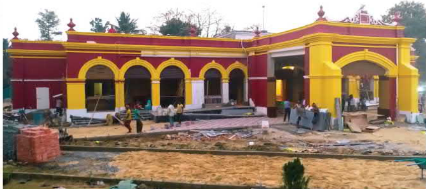
(Exterior work of the museum)
